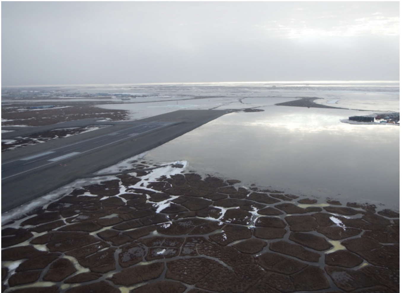
Southeast end Deadhorse runway flooding resulted from aufeis on the Sag River. (J.Organek ADOT)
