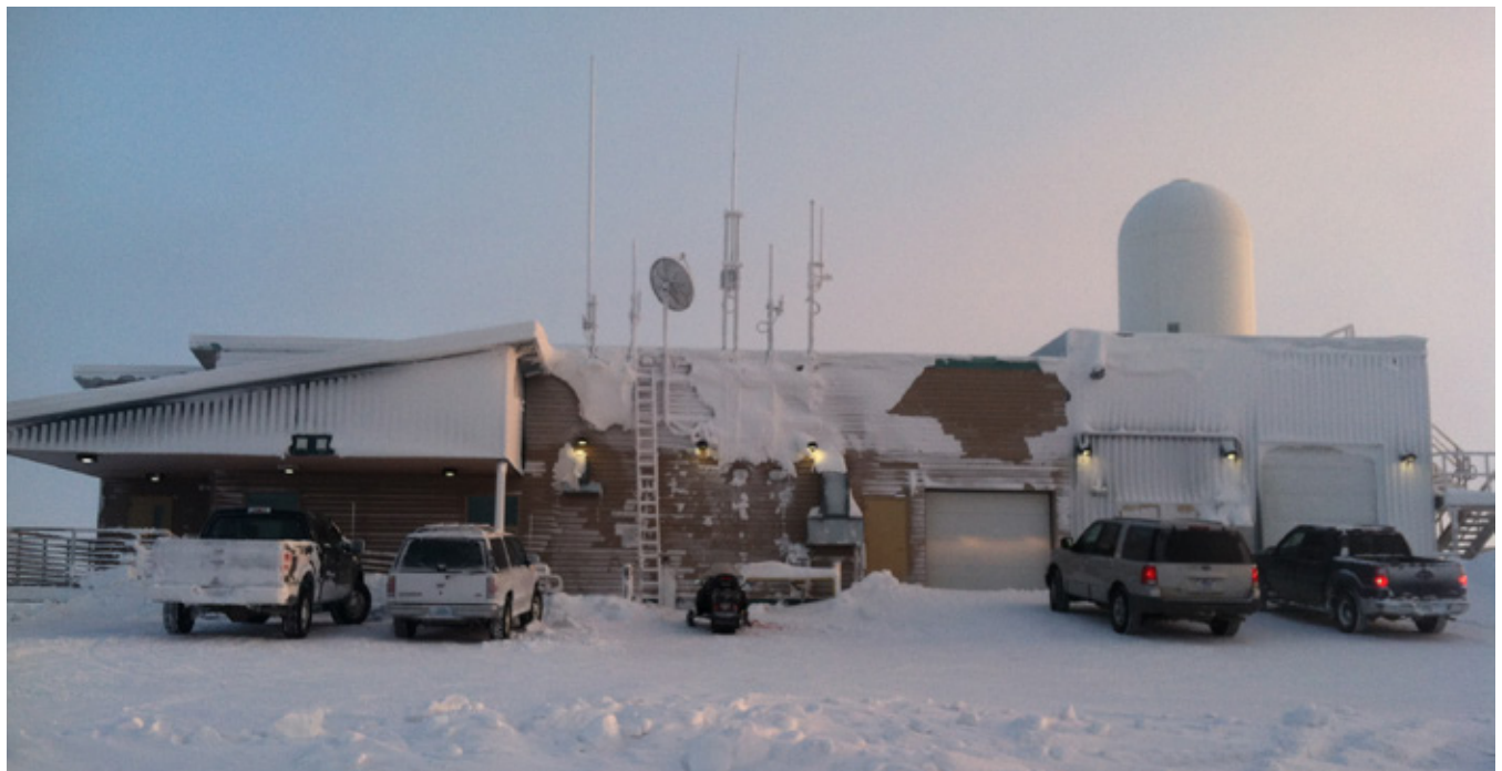
Weather Service Office in Barrow with dome housing radiosonde tracking antenna. (NOAA)
