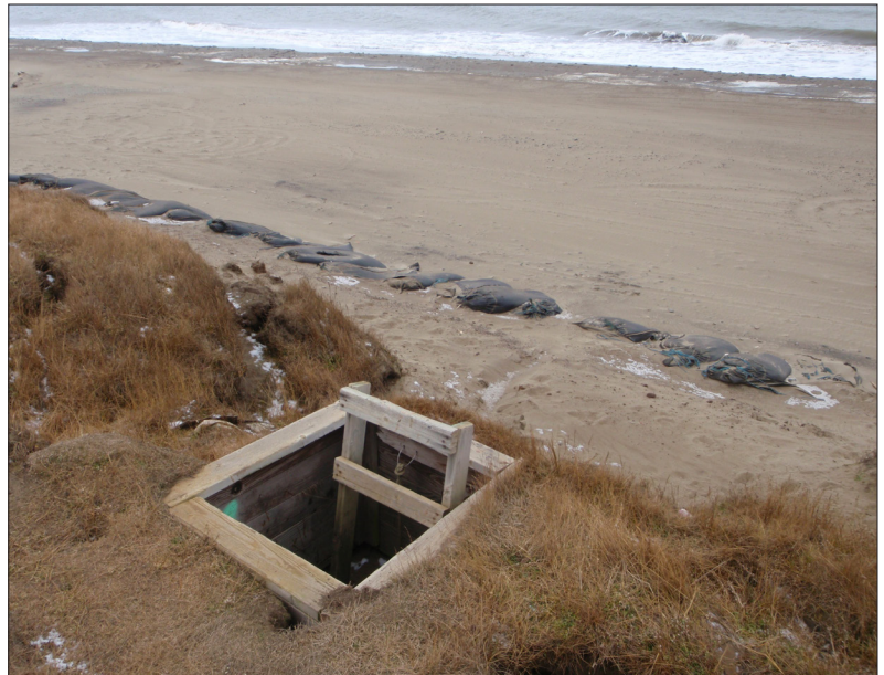
Ice cellar near Wainwright, Alaska, is threatened by permafrost degradation and increasing coastal inundation. (Li Erikson, USGS)
