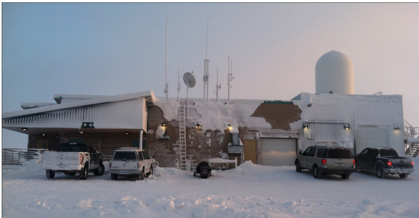
Weather Service Office in Utqiagvik with dome housing radiosonde tracking antenna. (NOAA)
