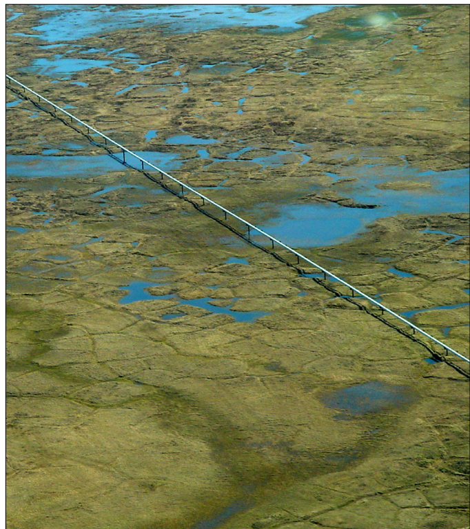
Pipeline over tundra on the north slope. (USGS)
