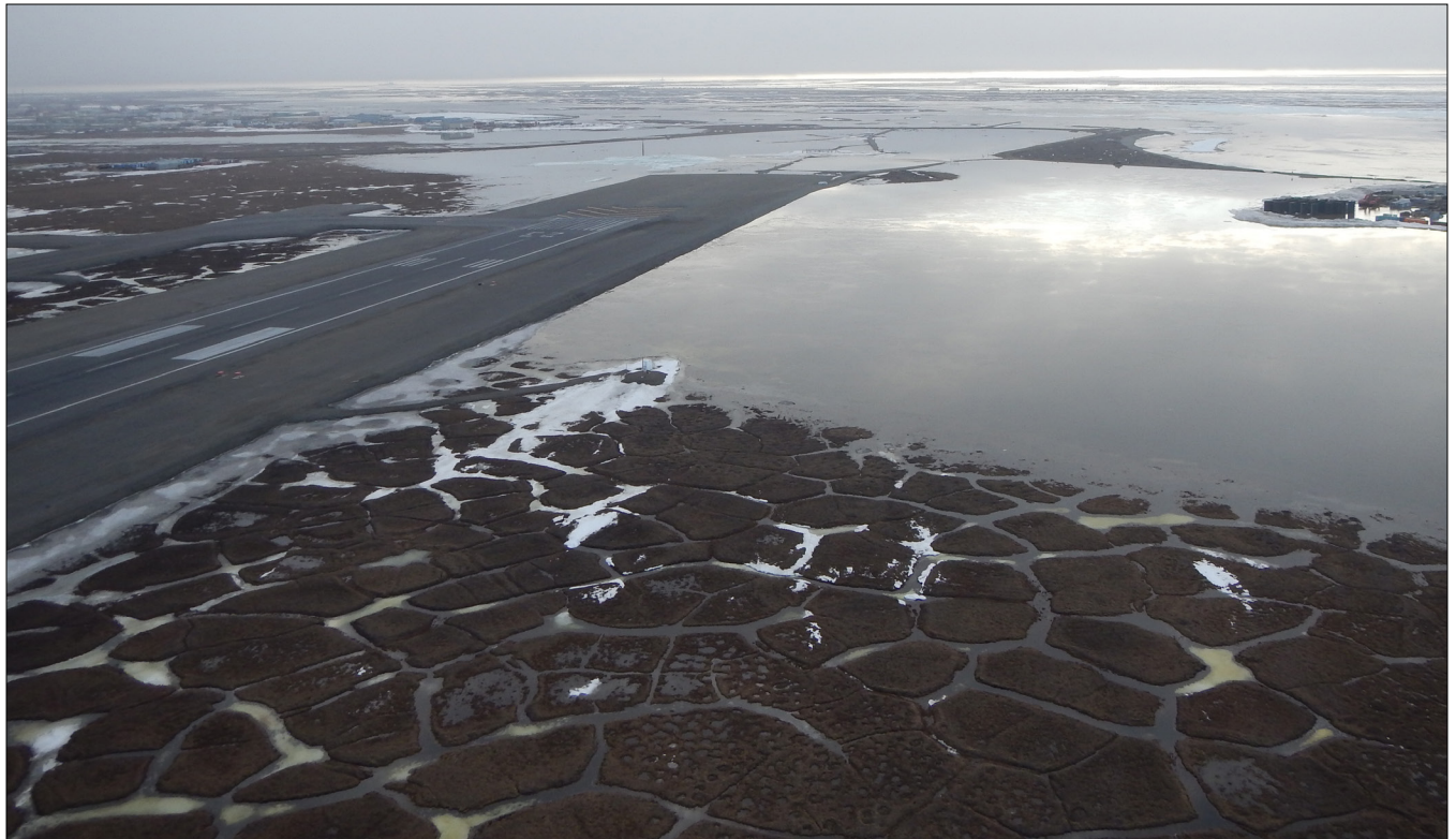
Southeast end Deadhorse runway flooding resulted from aufeis on the Sag River. (Jeff Organek/ADOT)
