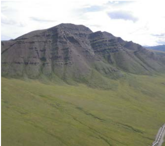
Land form varies from coastal plain to mountains along the pipeline corridor. (NSSI)
