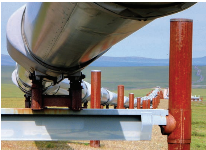
Trans-Alaska Pipeline (Doug Kane, UAF)
