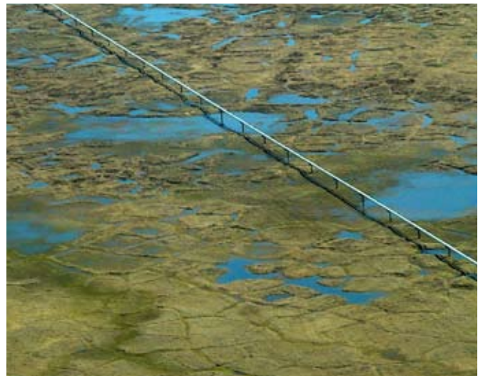
A roadless oil pipeline spans North Slope tundra. (USGS)
